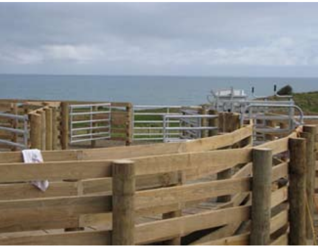
Paturau's new cattle yard under construction
