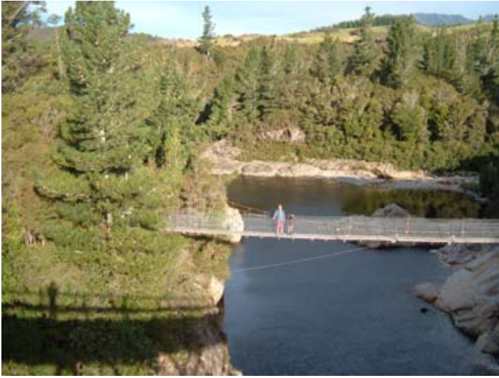
The historic swing bridge, built in the late 1860s and now extinct as a result of the 28th December flood
