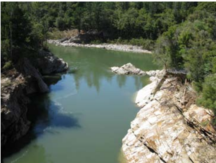
This photo, taken two days after the flood and again taken from the main bridge, shows the river almost back to its normal flow with the remains of the swing bridge against the right hand bank.
