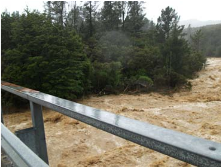
The river in full flood taken 8.45am; note the remains of the swing bridge, centre photo.
